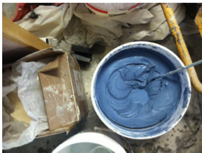
Site visit, April 17: Gray-blue plaster for the ceiling.
