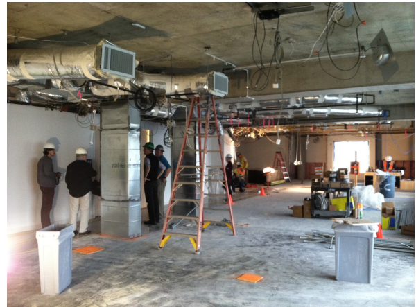
Construction of the Edith O'Donnell Institute's UTD headquarters on February 20, 2015.
